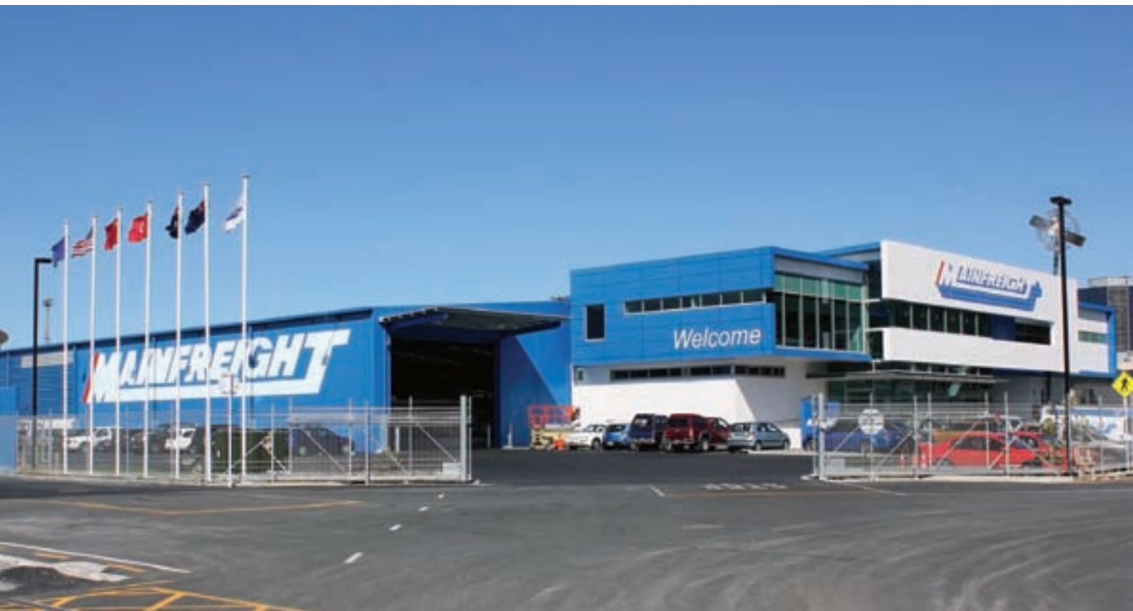
Mainfreight Terminal Wellington Rail Yards
